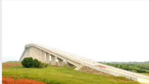
Long Slope Bridge
